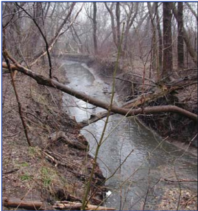
Existing highly erosive trench to pond photo by David S. Liebl
