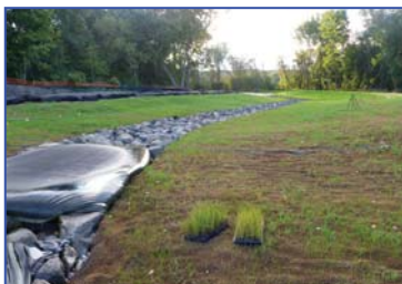
Construction: natural channel (left) and stilling pond (right).
