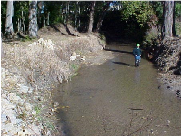
The Pheasant Branch stabilization project
